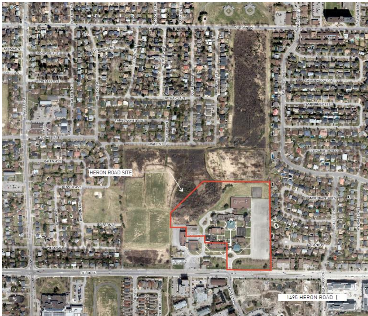
Figure 2: Aerial view of 1495 Heron Road and surrounding neighbourhoods
